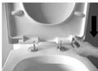
④ Install the toilet seat
