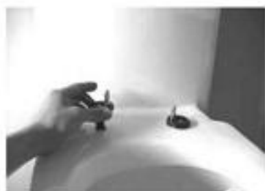
① Put the screw insert to the toilet hole
